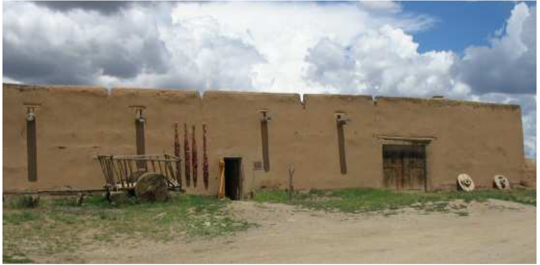
Entry Gate, Martinez Hacienda
