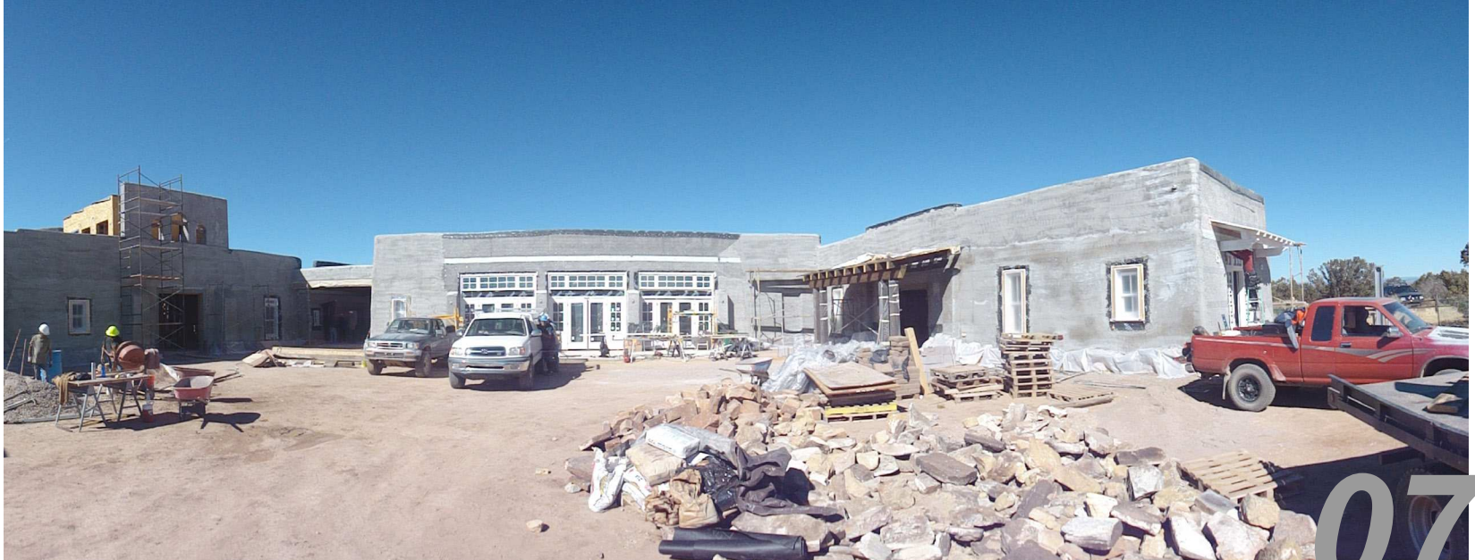
View of Courtyard looking North
