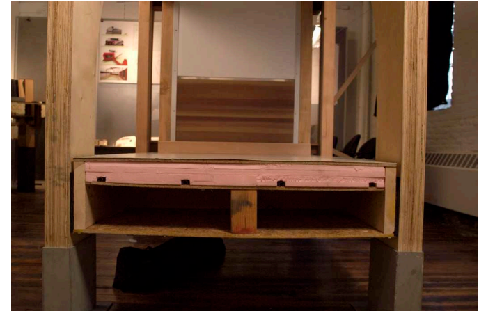
Floor Assembly of typical Rib-Panel Bay
