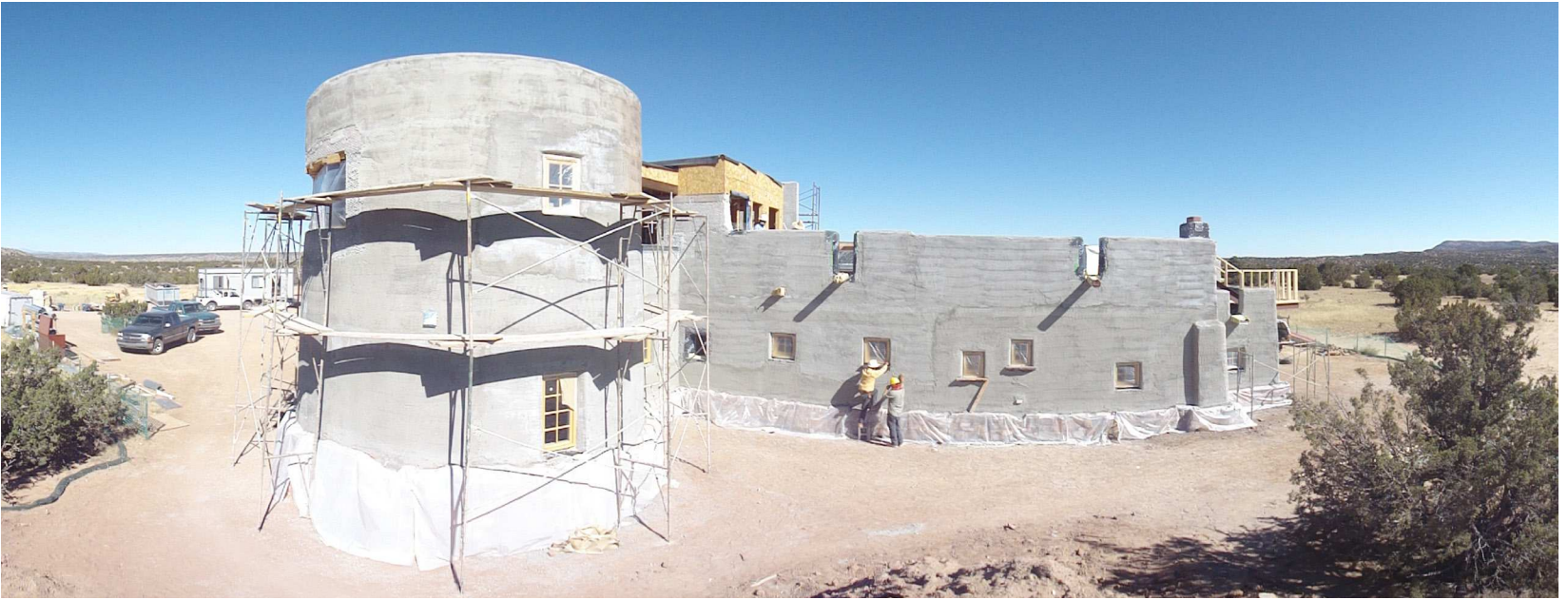
Construction of West Torreon
