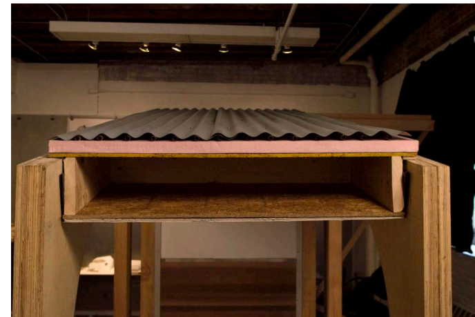
Roof Assembly of typical Rib-Panel Bay
